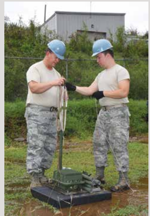
Master Sgt. David Fernelius, left, and Airman 1st Class David Zham, Joint Incident Site Communication Capability team members with the 151st Air Refueling Wing Communications Flight, erect an NVIS high-frequency antenna outside the Leonard B. Francis Armory in St. Thomas, U.S. Virgin Islands, Sept. 20, 2017. The Sept. 7 deployment of the Utah JISCC helped re-establish critical military and emergency, civil-service communications within areas of the U.S. Virgin Islands severely impacted by Hurricanes Irma and Maria.
